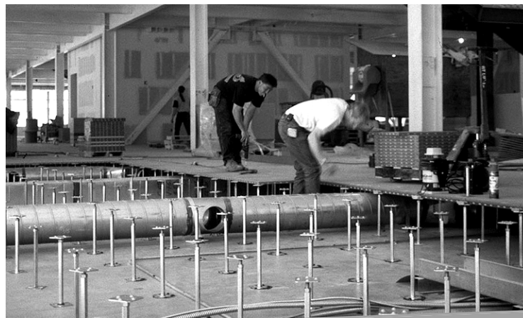
Figure 1 Raised floor installation, above ductwork and cabling in place. (Image: D. Lehrer)
